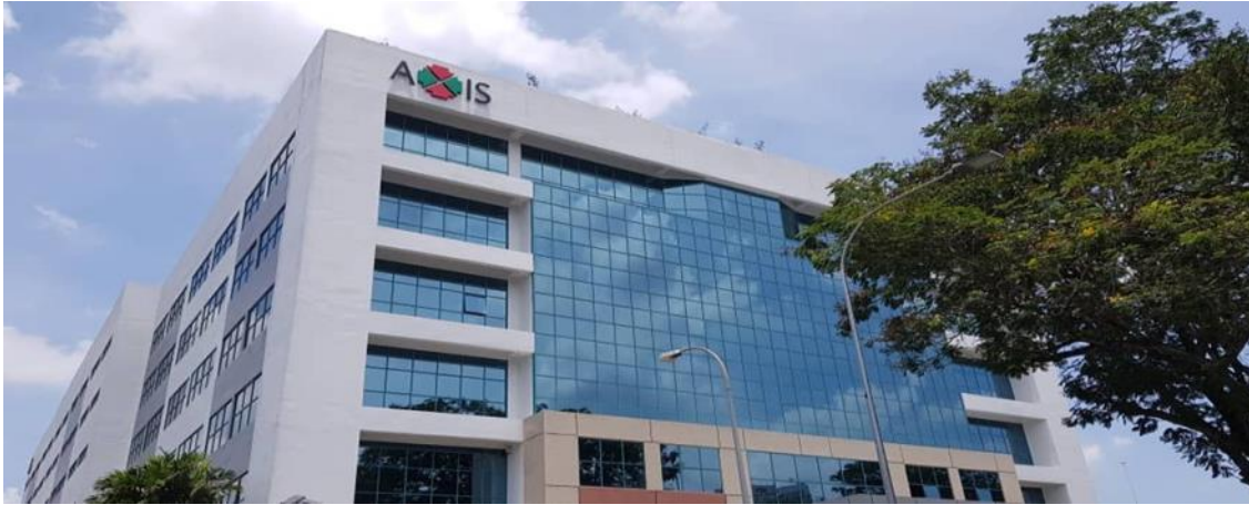
Wisma Academy Re-branding Signage: Front Facade
